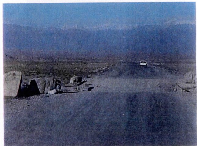
photo 7. Partially sunken bridge (16.1 km). Road surface drops approximately 8 inches to the bridge deck. Span approximately 10m. Overall, bridge in good condition.
